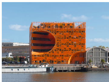
The Orange Cube (headquarters of Groupe Cardinal), Lyons, France - Photo © Roland Halbe
