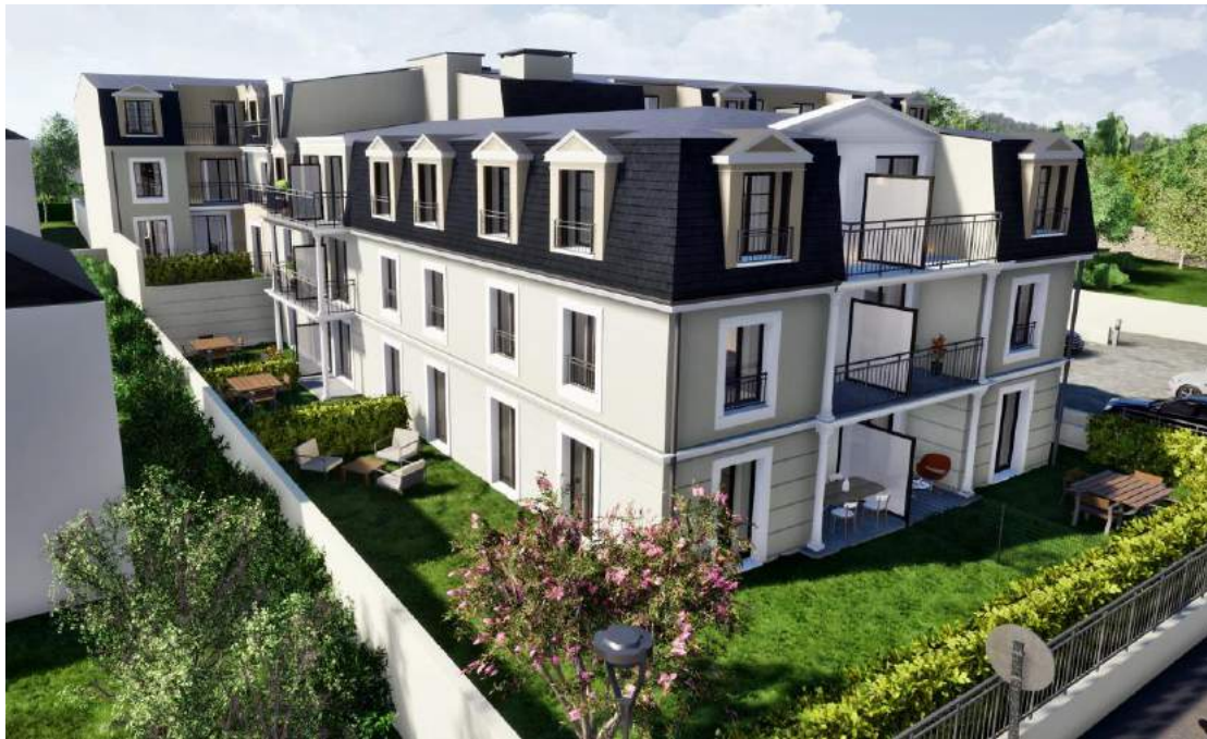
Construction of forty-five collective housing in Seine-et-Marne, France
