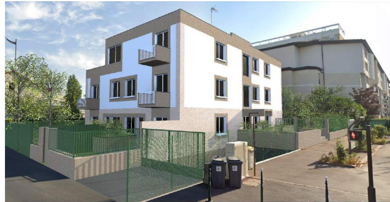
Renovation of an individual housing building in Reuil-Malmaison, France
